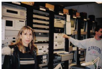
Ruba in the transmitting station/2002
